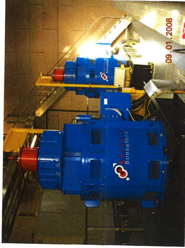
Head 7 meters, Output 2 x 450 kW, France
